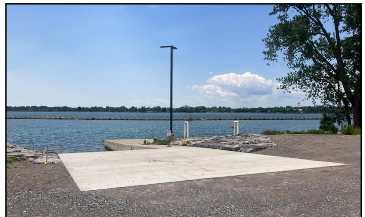
The new concrete pad at the top of the boat ramp.
