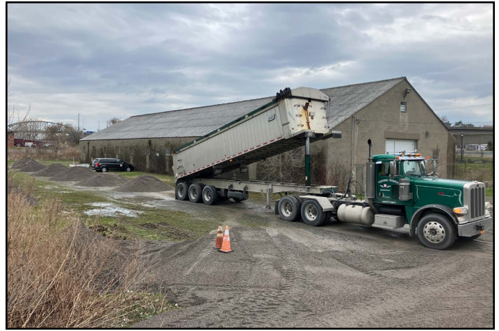
Delivering stone for the boat storage access road.
