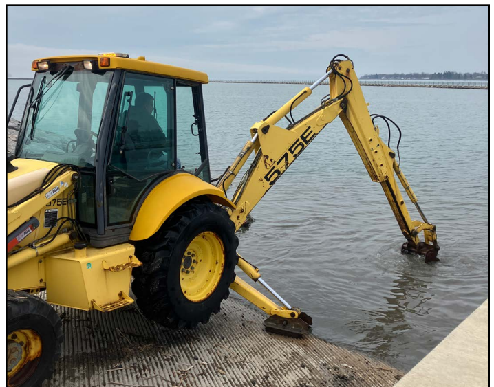
Clearing debris from the end of the boat launch.
