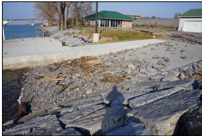
Stone deposited in the boat launch from the storm, filling most of the ramp with gravel of various sizes.
