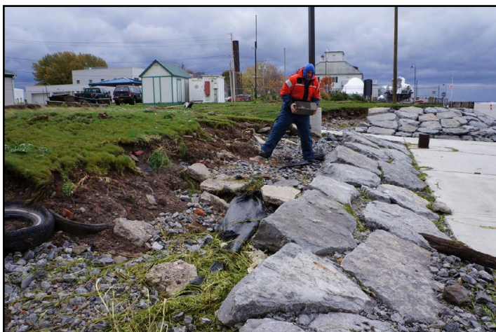
Brian Haas inspecting a section of shoreline with major erosion showing the loss of lawn from the high waters.
