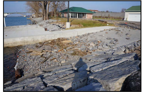
Stone deposited in the boat launch from the storm, filling most of the ramp with gravel of various sizes.
