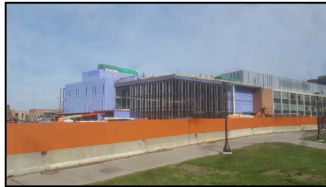
The south side of SAMC Phase 4.
