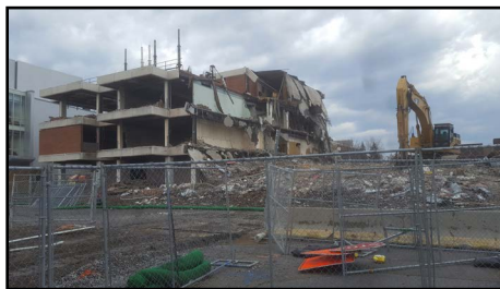
About half of the Science Building has been demolished so far.
