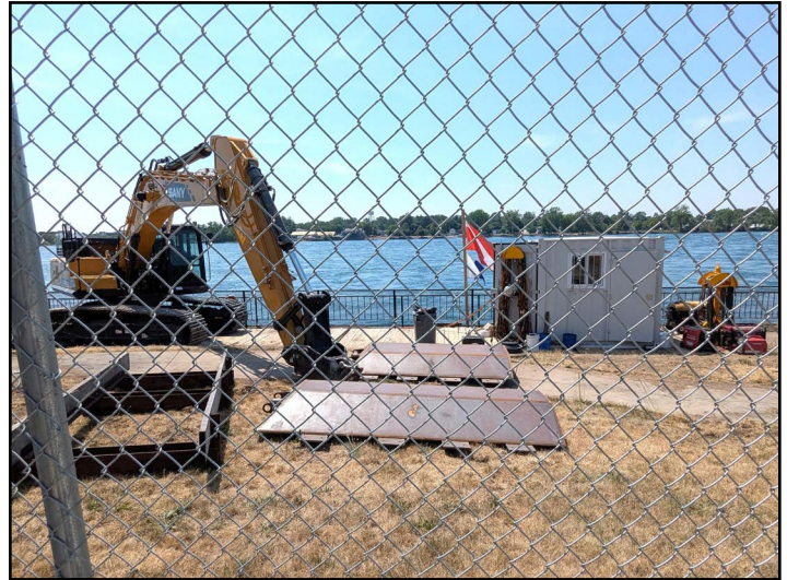
The baffles come in many sizes and shapes, and are being attached to the concrete wall by divers.
