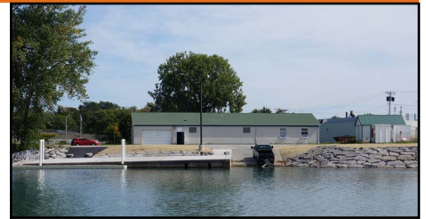
After: The ramp is steeper and has less obstructions around it. The dock has a nice concrete top and a floating dock with a ramp down to it. The shoreline is neatly wrapped with stone.
