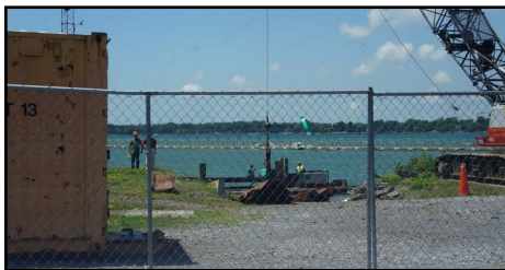
A crane was used to install the steel cofferdam.
