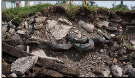
Before: The shoreline was made of a variety of fill, including tires.
