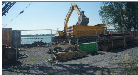
An excavator removes the old ramp and fill from the launch area.
