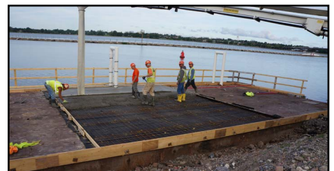
Concrete was poured onto the existing dock.
