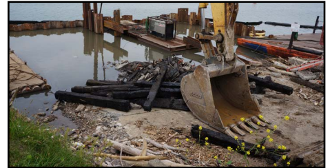
Before: There were also a lot of old dock pilings and cribbing below the water that had to be removed.
