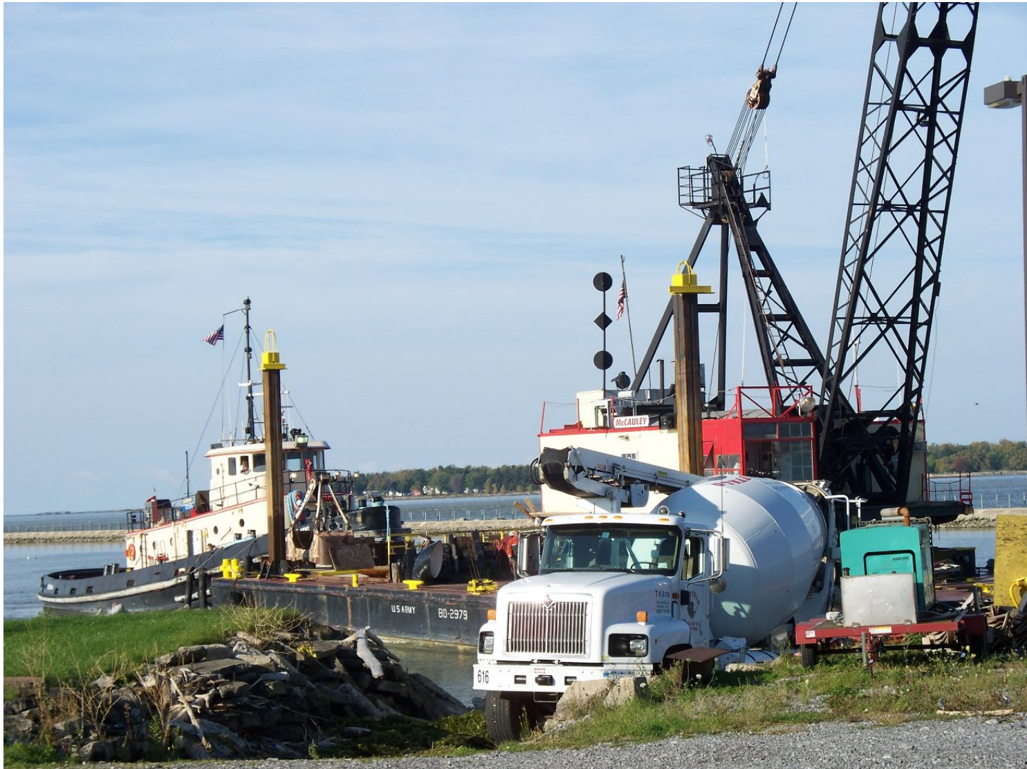
Army Corps Concrete deliveries for work on the break wall
