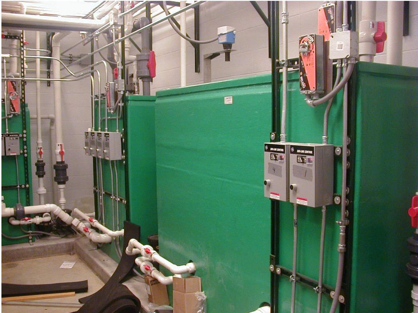
Holding tanks for three different temperatures of water for experiments
