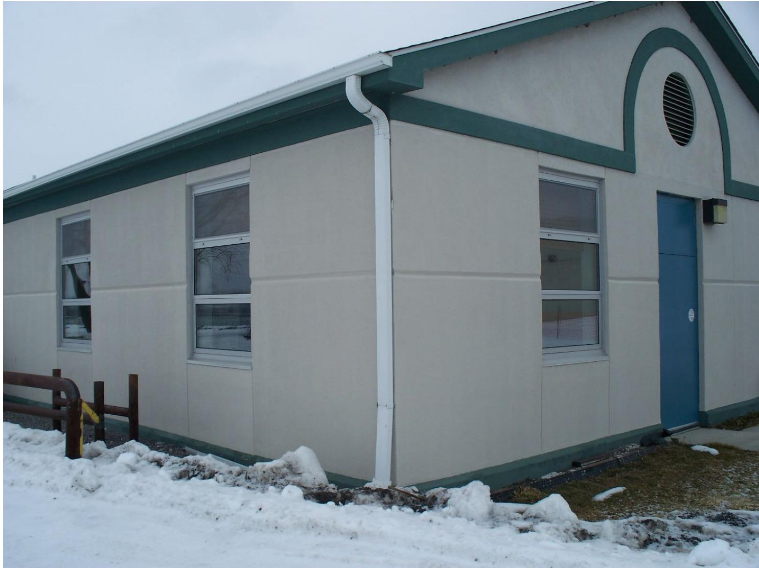
New windows at the Field Station for the main office
